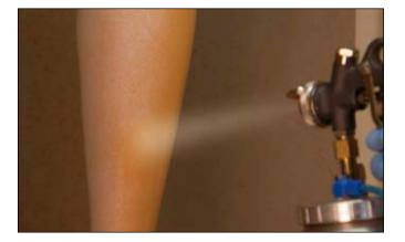
Apply a light coat of 635C3 Primer to the entire prosthesis (except the feet) at a pressure of 1.5 bar (primer does not have to be used up).
